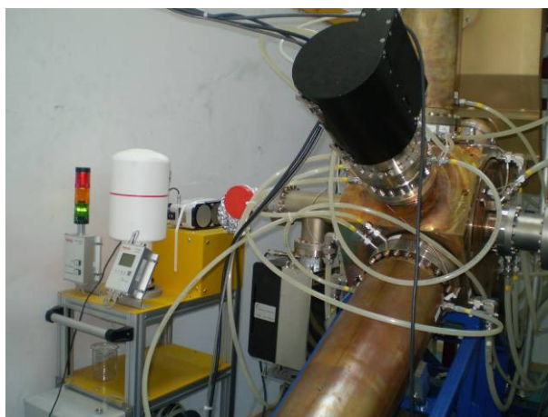
Fig.1 - ALBA SR cavity inside the bunker.
